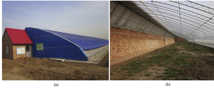
Fig. 1 – The overall appearance (a) and internal layout (b) of experimental Chinese Solar Greenhouse (CSG) located in Yangling, Shaanxi, China with dimensions 80 m long (E–W) and 10 m wide (S–N).
